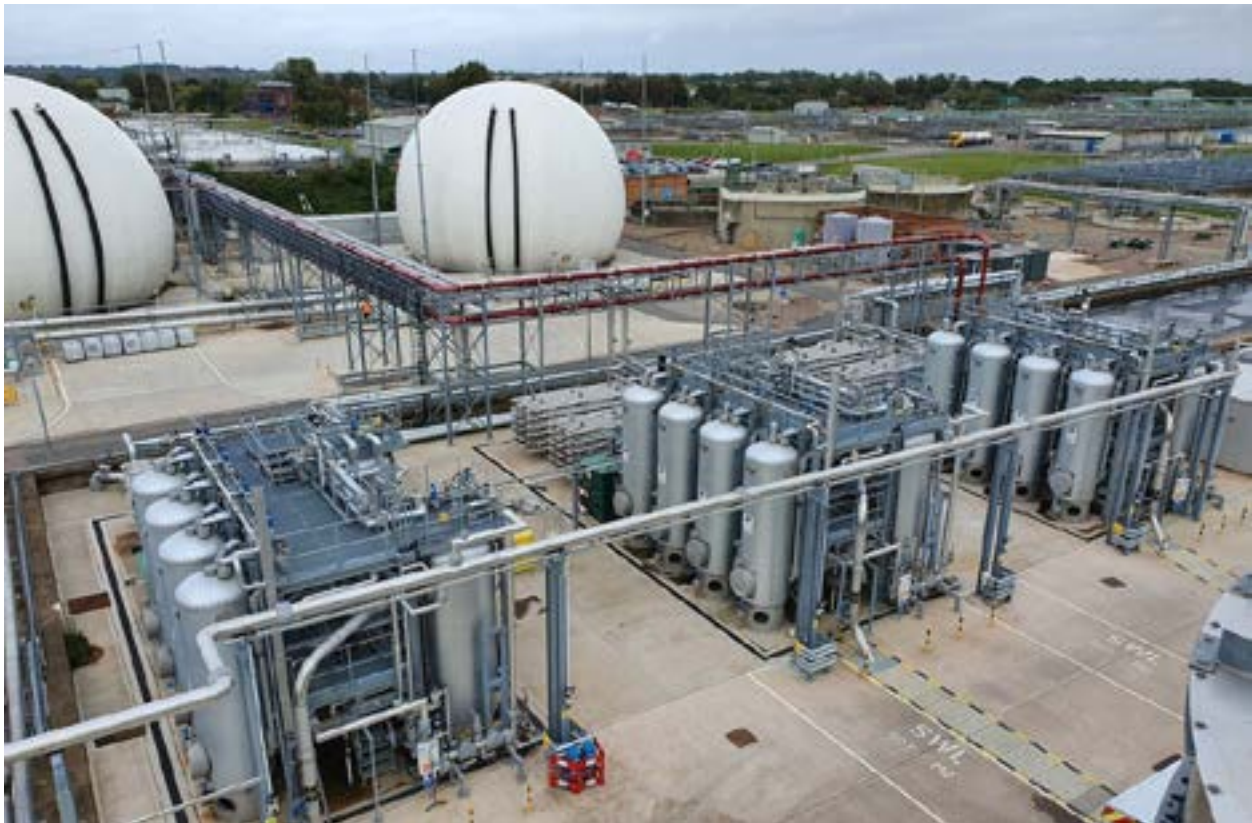
Figure 4: An illustration of a sludge treatment plant using THP and advanced anaerobic digestion. This plant treats 250 tonnes of sludge (on a dry basis) per day from a 500 MLD STP. Image Credits: Elliot Hobbs, Minworth STP, Birmingham, UK
